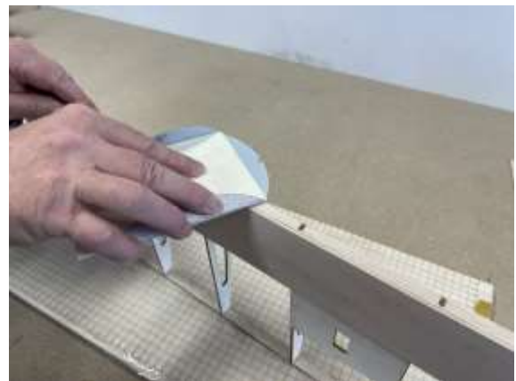
Sand wing flush at front.
