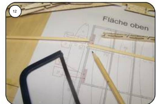
Cut the lower spar belt pine 2x4 mm according to the plan. One millimeter excess can't do any harm.
